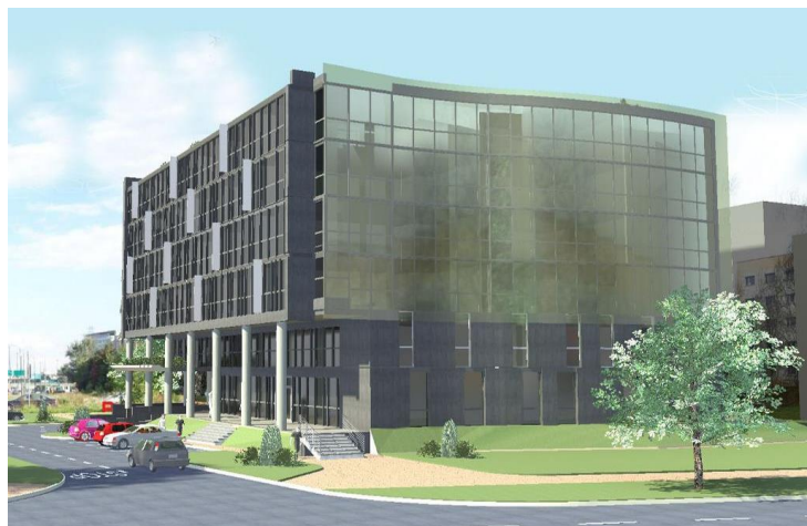
Sky Office Center, Warszawa
